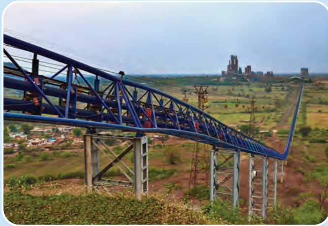
7.5 KM, 1500 MTPH, Pipe Conveyor at Manikgarh Cement, Unit-II, Gadchandur, Maharashtra for conveying Lime Stones
